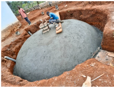
c) Fixed-dome biogas plant under construction
