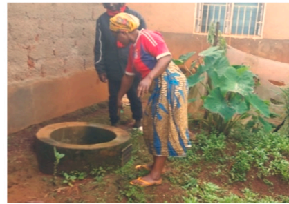
d) Underground domestic biogas plant
